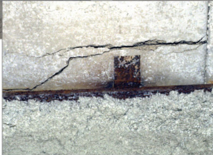
1st floor cored plank fractures
